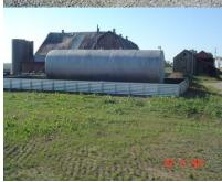
Ramsdell structures are a midpriced option. The company lets you assemble your own or they construct it for you. They are available in several shapes. The grain bin style looks good and could be torn down and moved to another site with the exception of the anchor posts.
