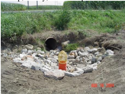
below-riser inlet showing restrictive orifice plate
