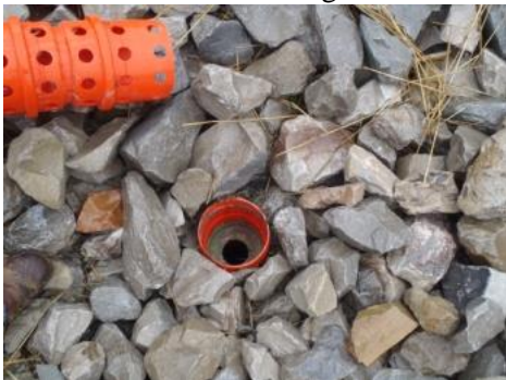
below-riser inlet showing restrictive orifice plate
