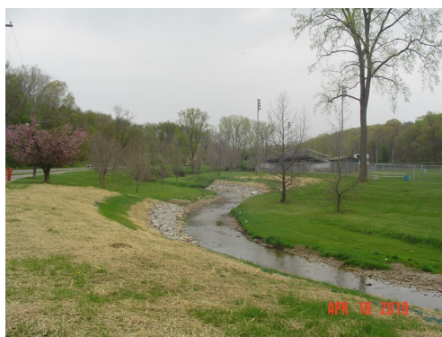
Lancaster High School Stream Bank Stabilization
