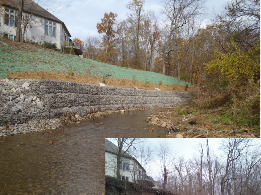
Above: Gabion basket wall with sloped and vegetated bank (before and after site)
