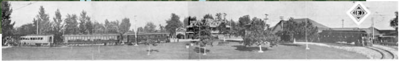
STATION, ENTRANCE, AND LOOP OF THE OHIO ELECTRIC RAILWAY AT BUCKEYE LAKE PARK.
