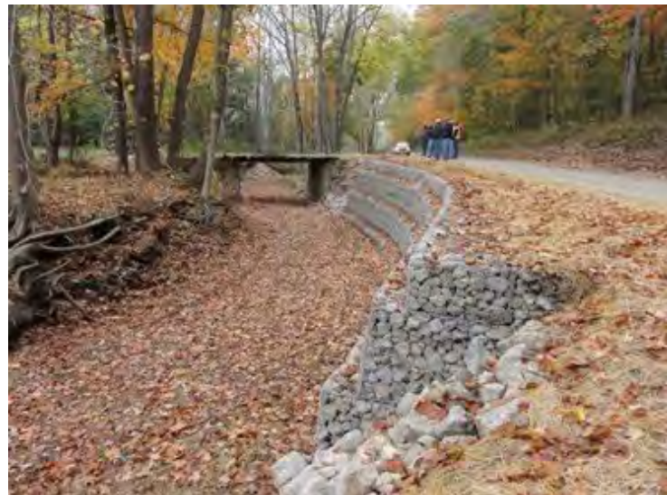
Below: 4 basket gabion wall along a road
