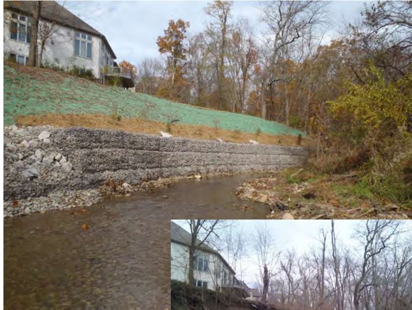
Above: 3 basket gabion wall with sloped and vegetated bank (before and after site)
