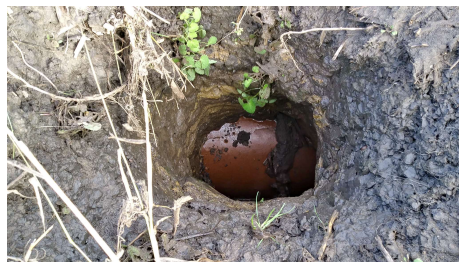
below-PVC outlet with animal guard and stone protection
