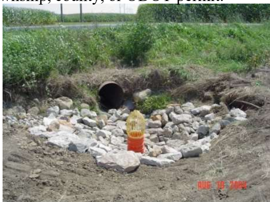
below-riser inlet showing restrictive orifice plate
