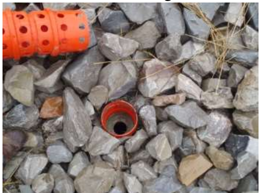
below-riser inlet showing restrictive orifice plate
