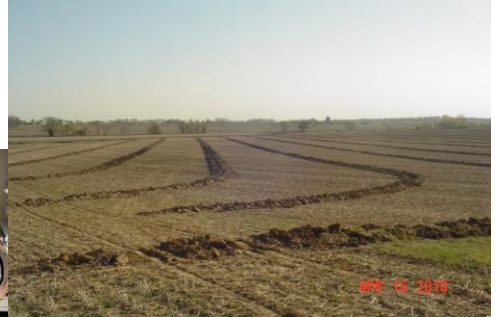
above-newly installed tile system in a farm field
