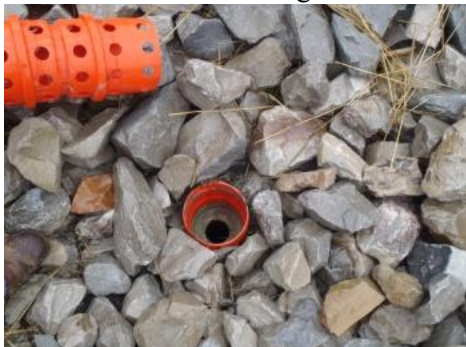
below-riser inlet showing restrictive orifice plate
