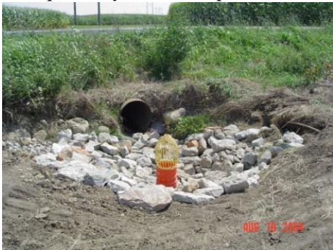
below-riser inlet showing restrictive orifice plate
